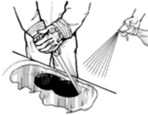
Hand Sawing Asbestos Cement Pipe
